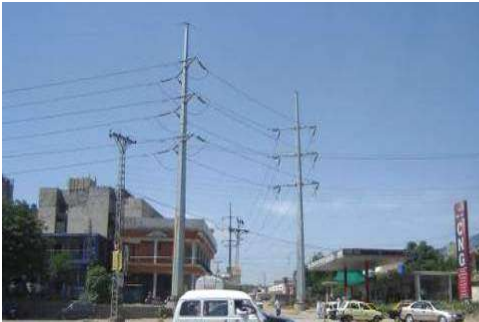
Figure 4.2: Korean Tubular Pole for city and high density populated areas
