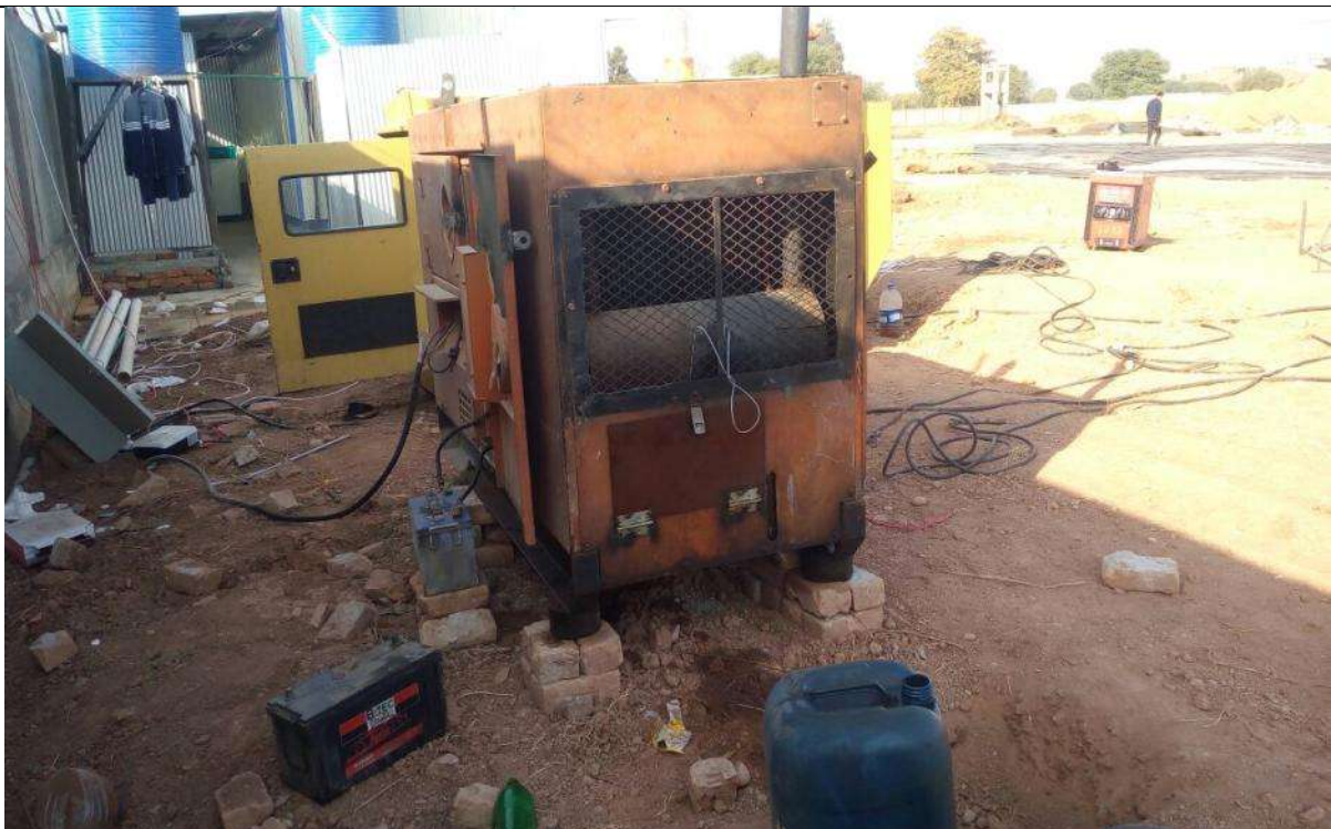
Oil spill and cables are scattered on the ground (Hazard for labors)
