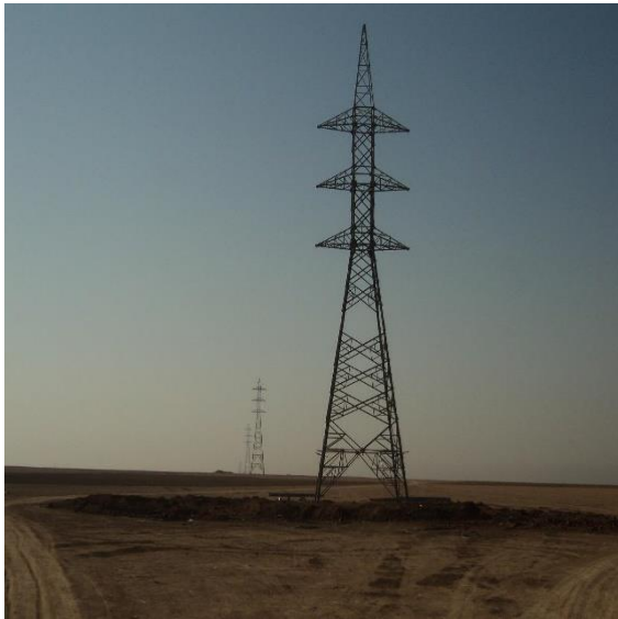
Figure 3.5: 132 KV Conventional Tower (Proposed)
