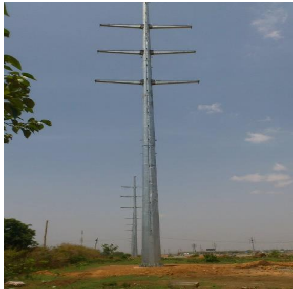
Figure 3.6: 132 KV Korean Tubular Pole
