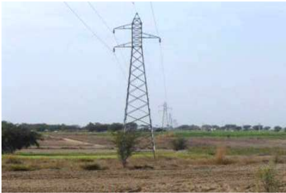
Figure 4.2: Typical Tower 66 KV for cultivated & barren Land.
